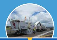
"With 3D mill and 3D paving controls from Trimble, we were able to lay 5,000 tons of asphalt to grade and slope per night, in a 12-hour shift compared to 2,000 or 2,500 tons per shift, on other jobs."
