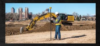
The Trimble Siteworks Positioning System for Construction Surveyors is comprised of the SPS986 or SPS785 GNSS Smart Antenna, the TSC7 Controller or T7 Tablet and Siteworks Software. It enables construction surveyors to work with complex 3D models, collect large data sets faster, visualize complex 3D models more easily and work day or night efficiently.
